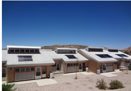
The Chuska Apartments in Gallup, NM provide transitional housing for homeless families. The NMCEH helped our member agencies CARE66 and Supportive Housing Coalition of New Mexico develop Chuska by providing technical assistance.
